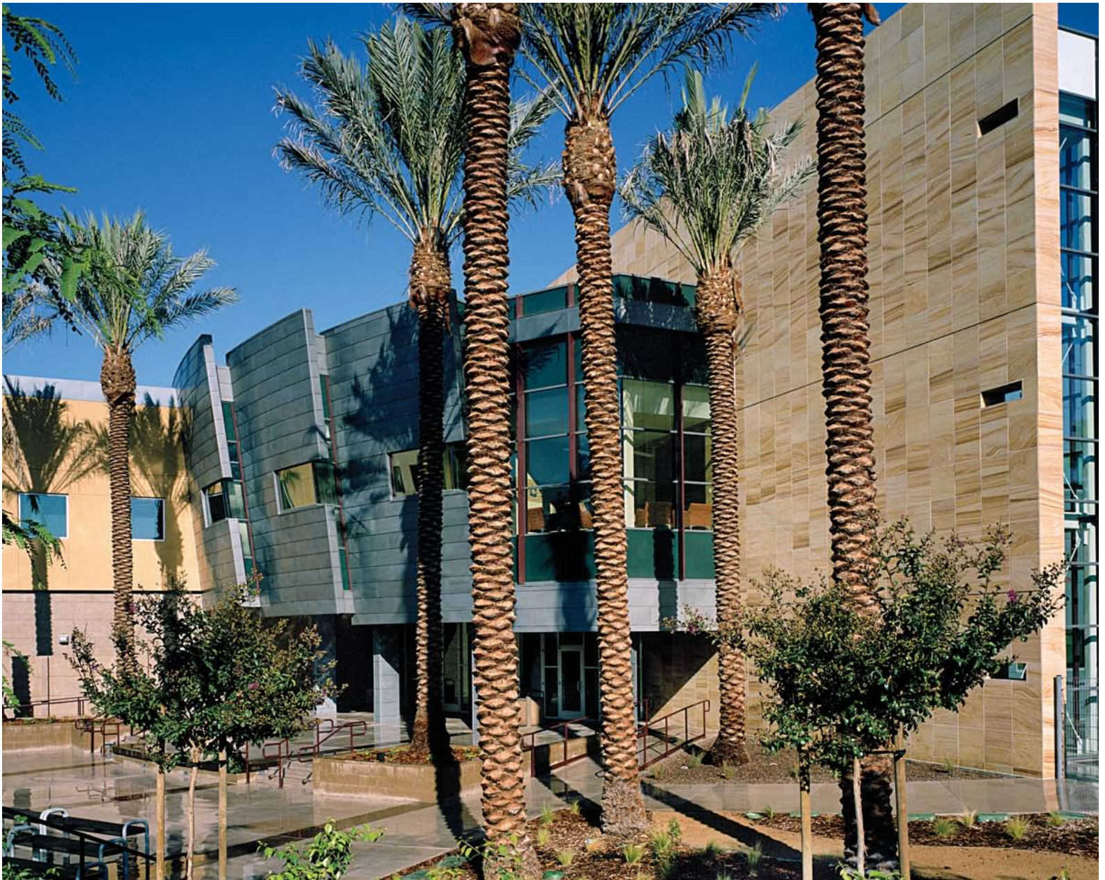
Cymer Office Building, San Diego, California
